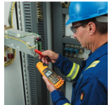
Measure process and other automation 4 to 20 mA signals without breaking the loop.
