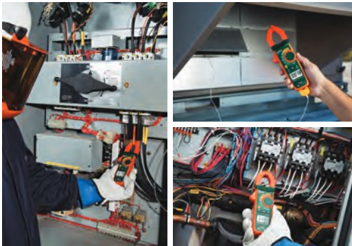
Troubleshoot current output on an electrical panel, verify Temperature output on HVAC units, and quickly detect live voltages with built-in Non-contact Voltage Detector.
